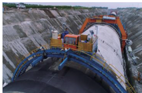
Fig. 5 Coating robot in operation
